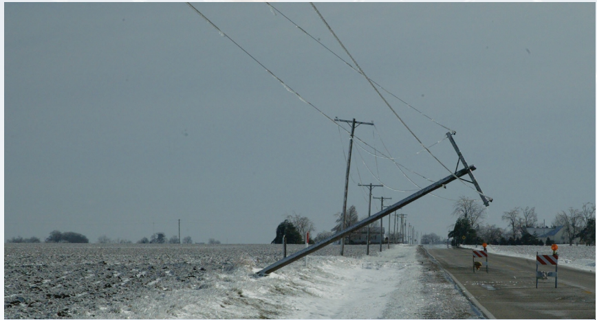
Ice buildup on power lines and poles, plus high winds, can cause galloping lines and poles to fall.
