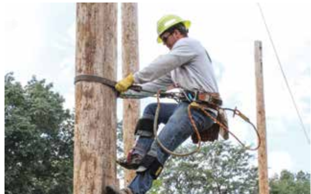
Apprentice Dalton Brown placed third in the individual apprentice H-structure event.
