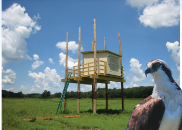
Shelby Electric Cooperative donated poles and labor to help build hacking stations like this one (photo above) and nesting platforms (photo below) at various spots on Lake Shelbyville.
